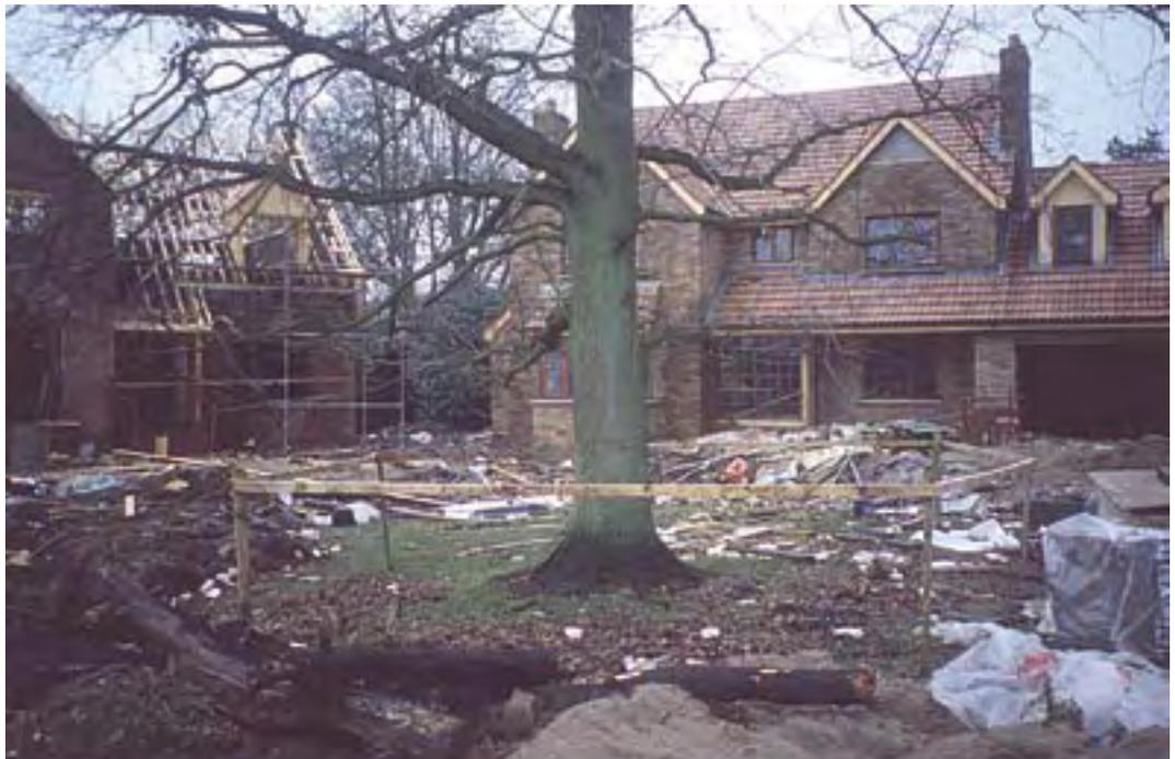
Inadequate fencing, debris and building materials under crown spread
