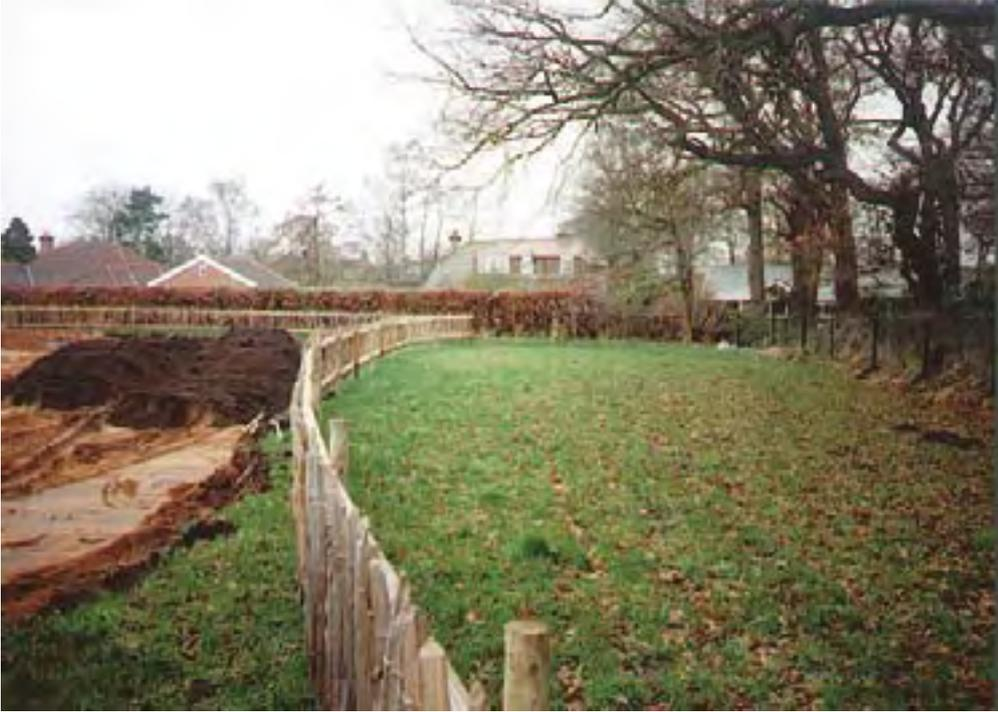
Erect temporary fencing around trees to be retained at the outer limits of the crownspread or at a distance of half the height of the tree, whichever is greater. Fencing should be at least 1.2 metres high cleft chestnut pale (or alternatively chain link), well braced to resist impacts.
