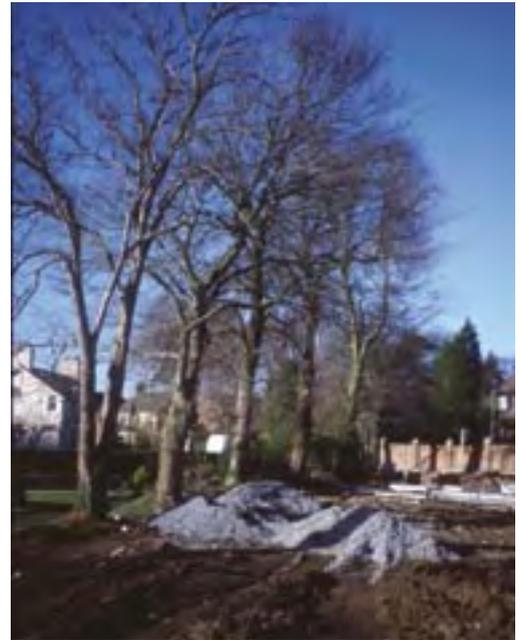
Inappropriate stockpiling of materials within crown spread
