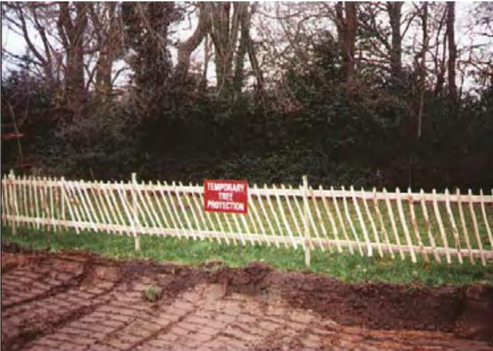
Ensure that the fencing is maintained during development and that all staff and contractors know the ground within the fenced area is protected. Attaching warning signs to the temporary fencing can also be helpful.
