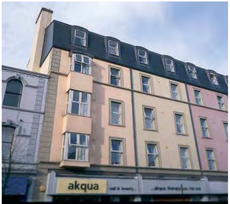
Successful provision of residential accommodation over shops. Londonderry
