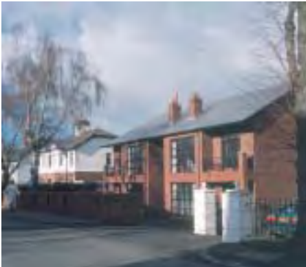
New housing integrated into the established urban environment. South Belfast
