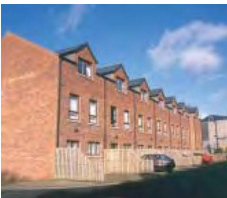
Rear courtyard car parking. South Belfast
