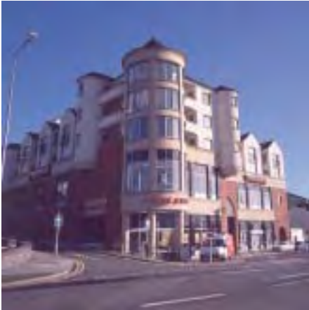
Mixed use development integrated with the surrounding community. Enniskillen, County Fermanagh
