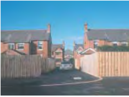
Access to backland development impacting on streetscape. East Belfast
