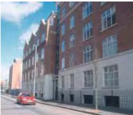
Semi-basement car parking. Belfast City Centre
