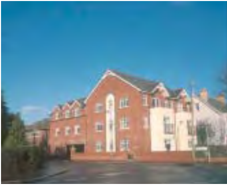
Demolition and redevelopment of a corner site. East Belfast
