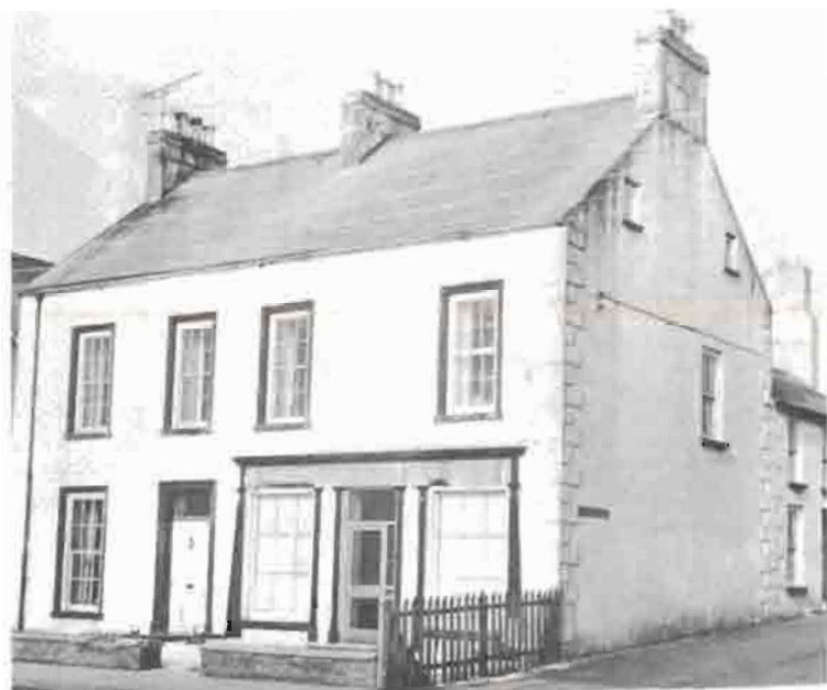
3. Nos. 19-21 Marine Road (Lanktree's House)
