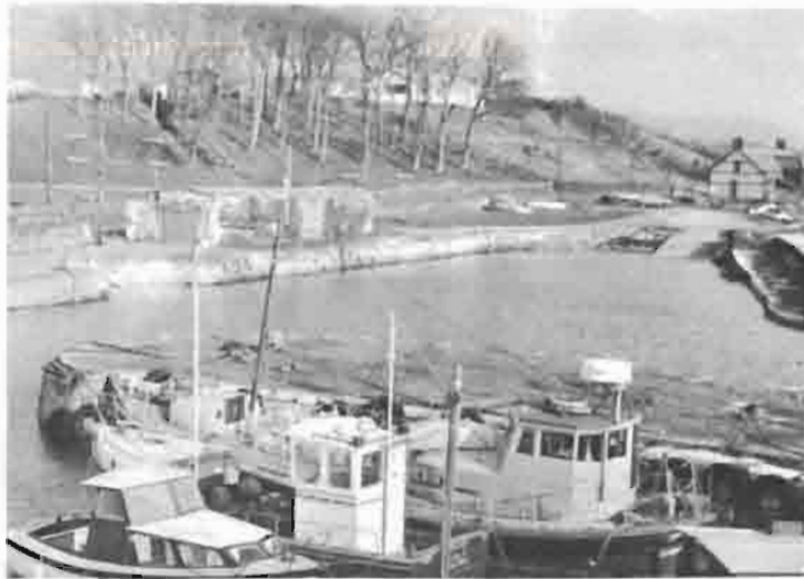
1. Harbour Road from the South Pier
