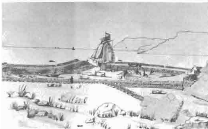
2. Carnlough Harbour Construction 1853--55
