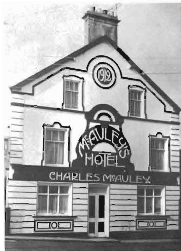
2. Nos. 2-4 Bridge Street (C McAuley's Hotel)
