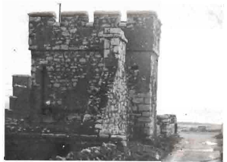
2. Eastern Tower Staircase, Harbour Road
