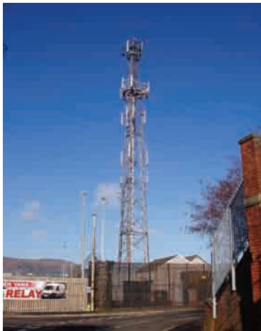
A Lattice structure located within an industrial area
