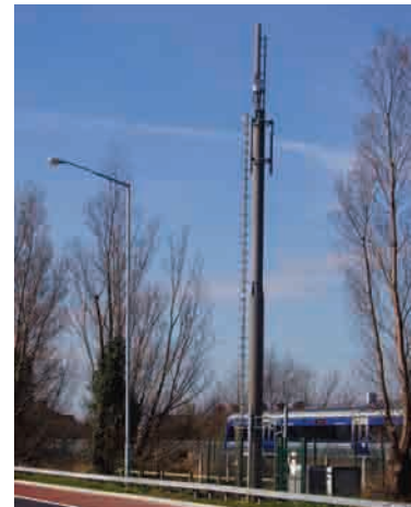
A mast located between a Dual Carriageway and a railway line
