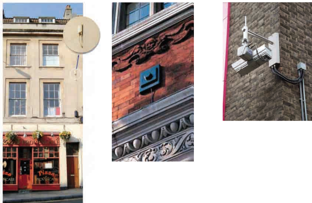
Examples of well integrated small scale antennas.
